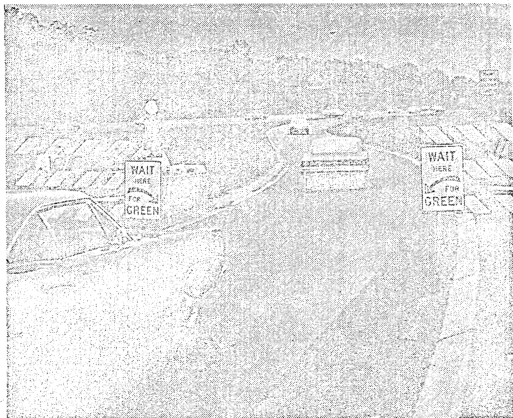
NEW FLASHING SIGNALS CONTROL MERGING TRAFFIC Experimental setup on Interstate 35E ramp in St. Paul
