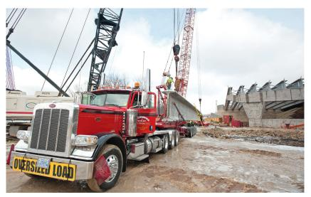
A large I-beam girder is unloaded from a truck with appropriate red flags and "Oversized Load" banner. Each governing authority that manages roadways along a hauling route may have a different permit application process and different signage and flagging requirements.
