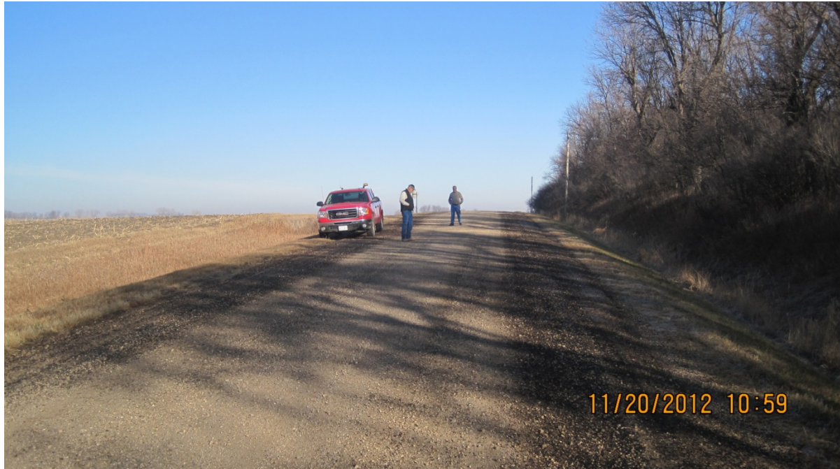
Figure 5 Jackson Co. Looking up grade on 520th Ave. from CR 81 1 to 1 blend
