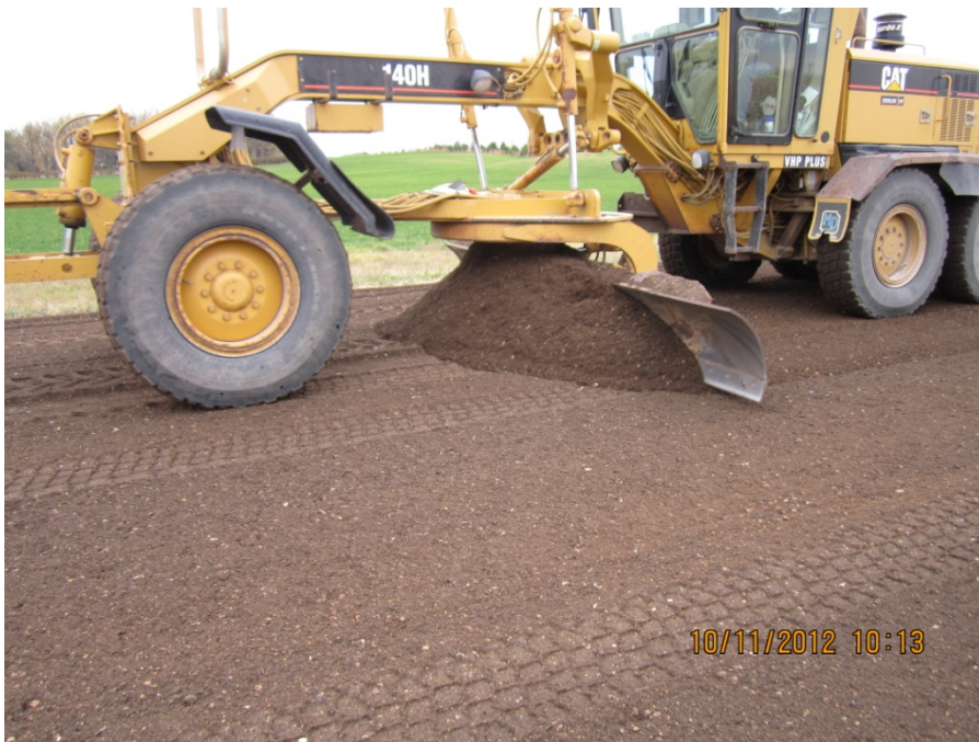
Figure 2 Jackson Co. shaping of 4/10 blend on CR 70
