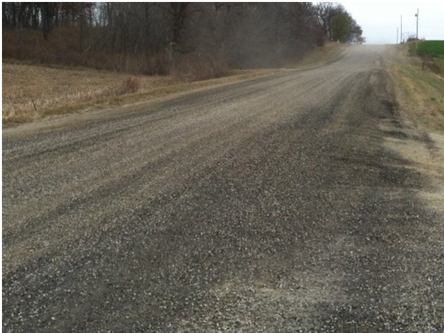
Figure 7 Goodhue CR 52 Finished blend of TOSS and Cl. 6
