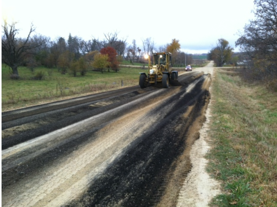
Figure 6 Goodhue CR 6 placing shingles on Cl 6 limestone
