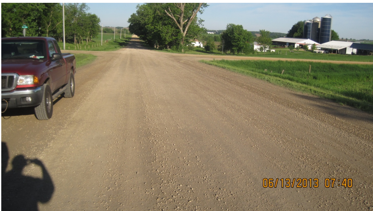
Figure 3 Goodhue County Shingle Section
