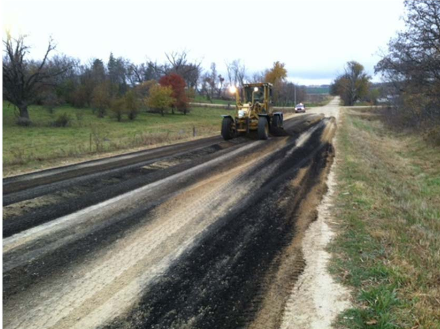
Figure 2 – Test Section Construction in Goodhue County
