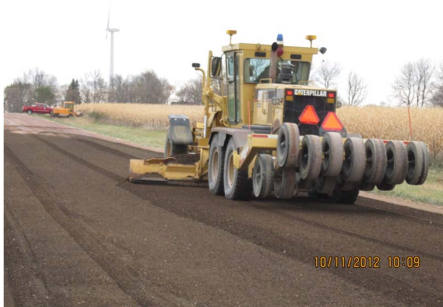
Figure 1 – Test Section Construction in Jackson County
