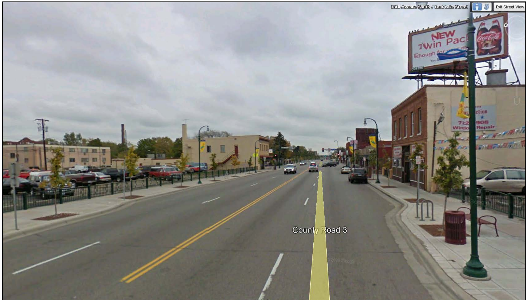
Figure 4.15: East Lake Street Cross-Section near 17 th Avenue After Reconstruction Showing Curb Extensions and Parking Lanes
