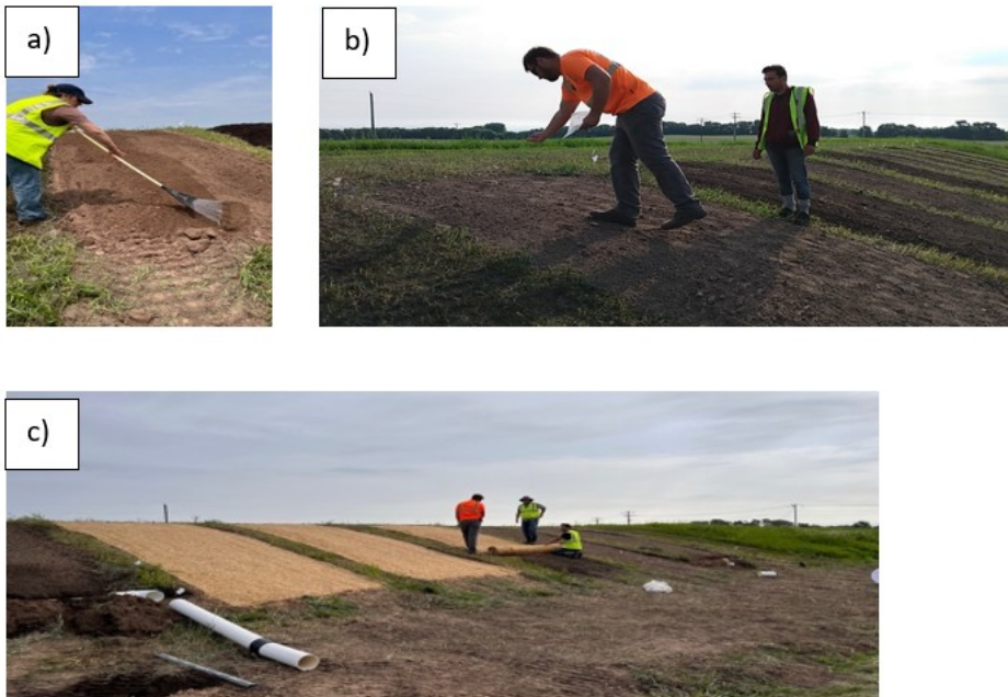
Figure 6.6 (a) Raking operation to create seed-bed contact, (b) distribution of seed mix through hand-broadcasting, and (c) application of erosion control blankets.
