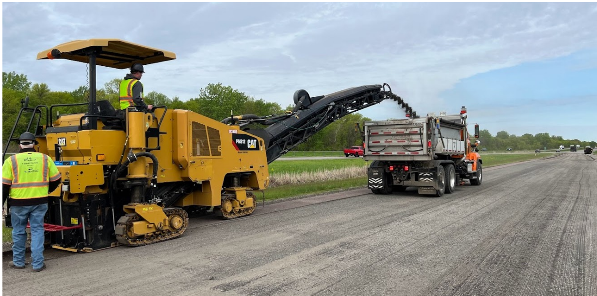
Figure 4-2. Milling Operation at MnROAD Research Facility in May 2022
