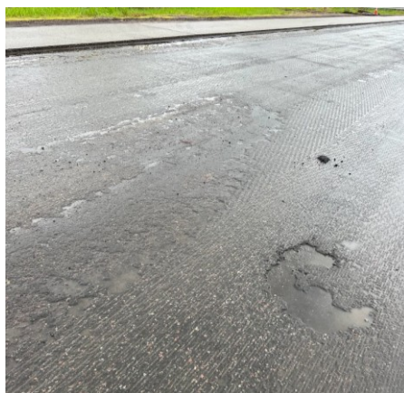
Figure 4-20 Mid-layer Delamination in MnROAD Cell 16 Driving Lane
