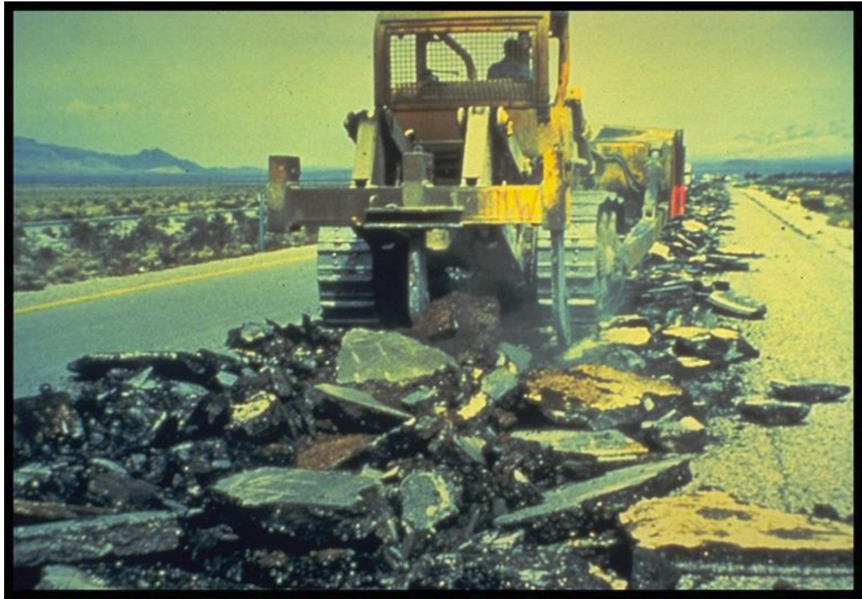
Figure 2-1 Dozer with Tipper-Tooth (Kandhal and Mallick, 1997)
