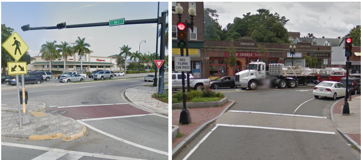
Figure 9. Examples of textured crosswalks at CRTs [3].
