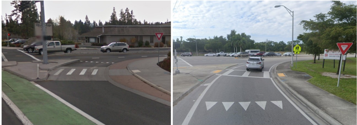
Figure 8. Example of advance yield markings at CRTs [3].
