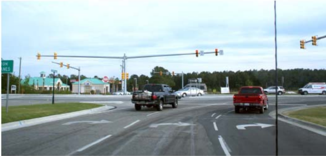
Figure 30: Signal Pole Locations on the Minor Approaches of an RCI on US-17 in North Carolina
