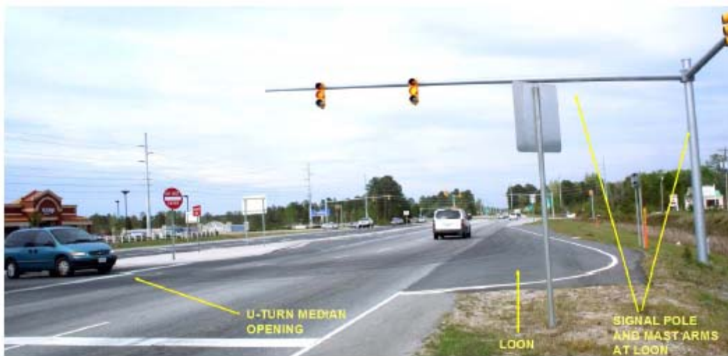
Figure 29: Median U-Turn Crossover Signal Pole Locations at an RCI in North Carolina
