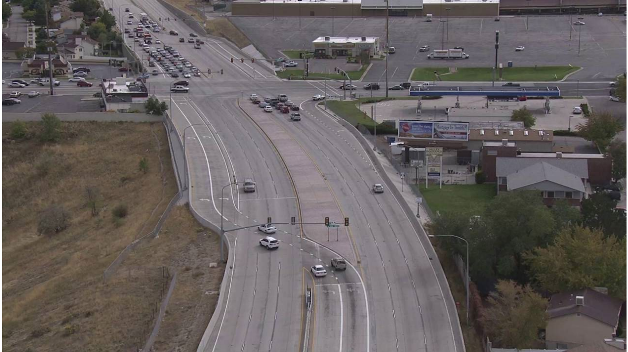
Figure 4.1: Displaced left-turn intersection
