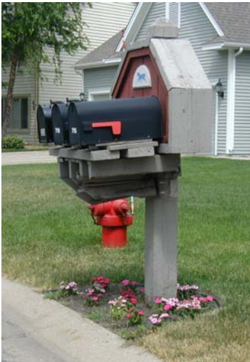
Example of Community Mailboxes Where Paper Boxes Were Struck by Winter Maintenance Equipment (too low and forward of back of curb)
