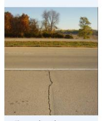
The use of a performance test in material specifications could help prevent the most common type of pavement distress in Minnesota—cracking caused by low temperatures.
