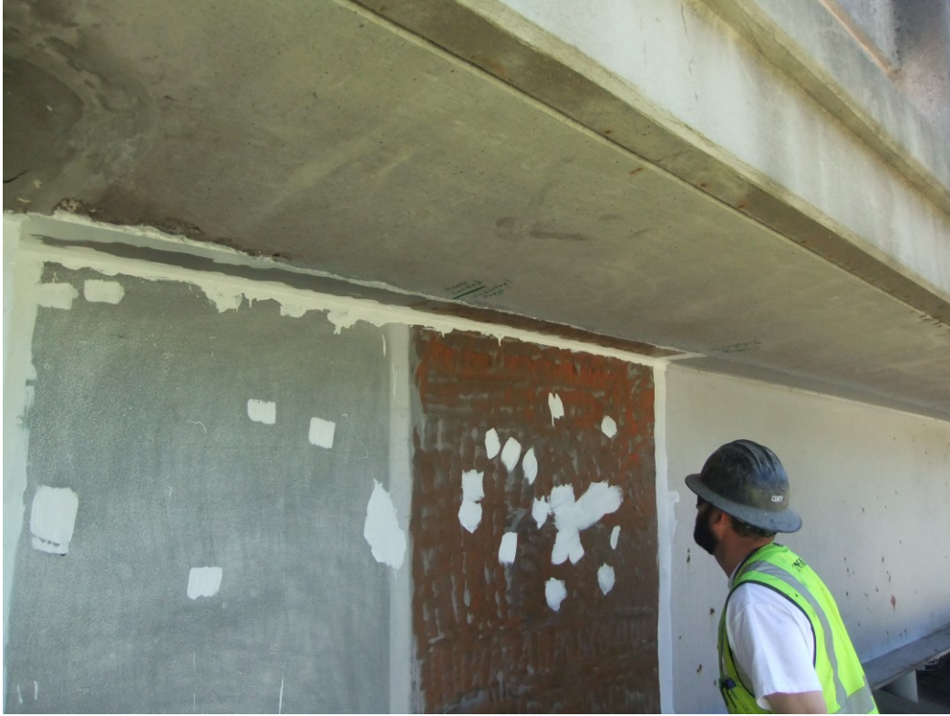
Figure 4.14 Test Location 5 Prime Coat Application
