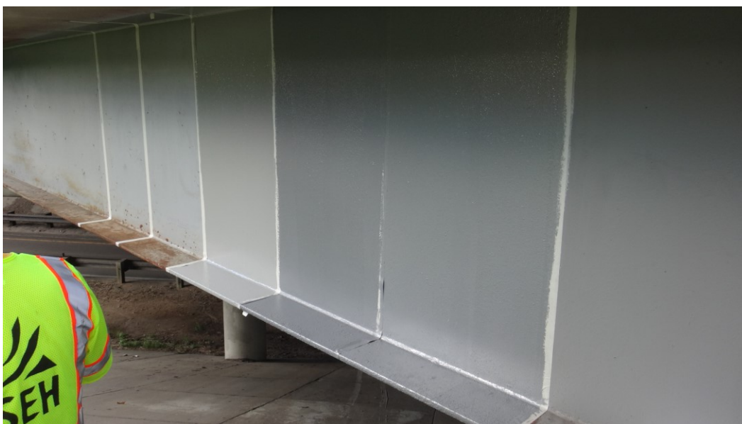
Figure 8.8 Additional Test Patch Location C - Coating Application
