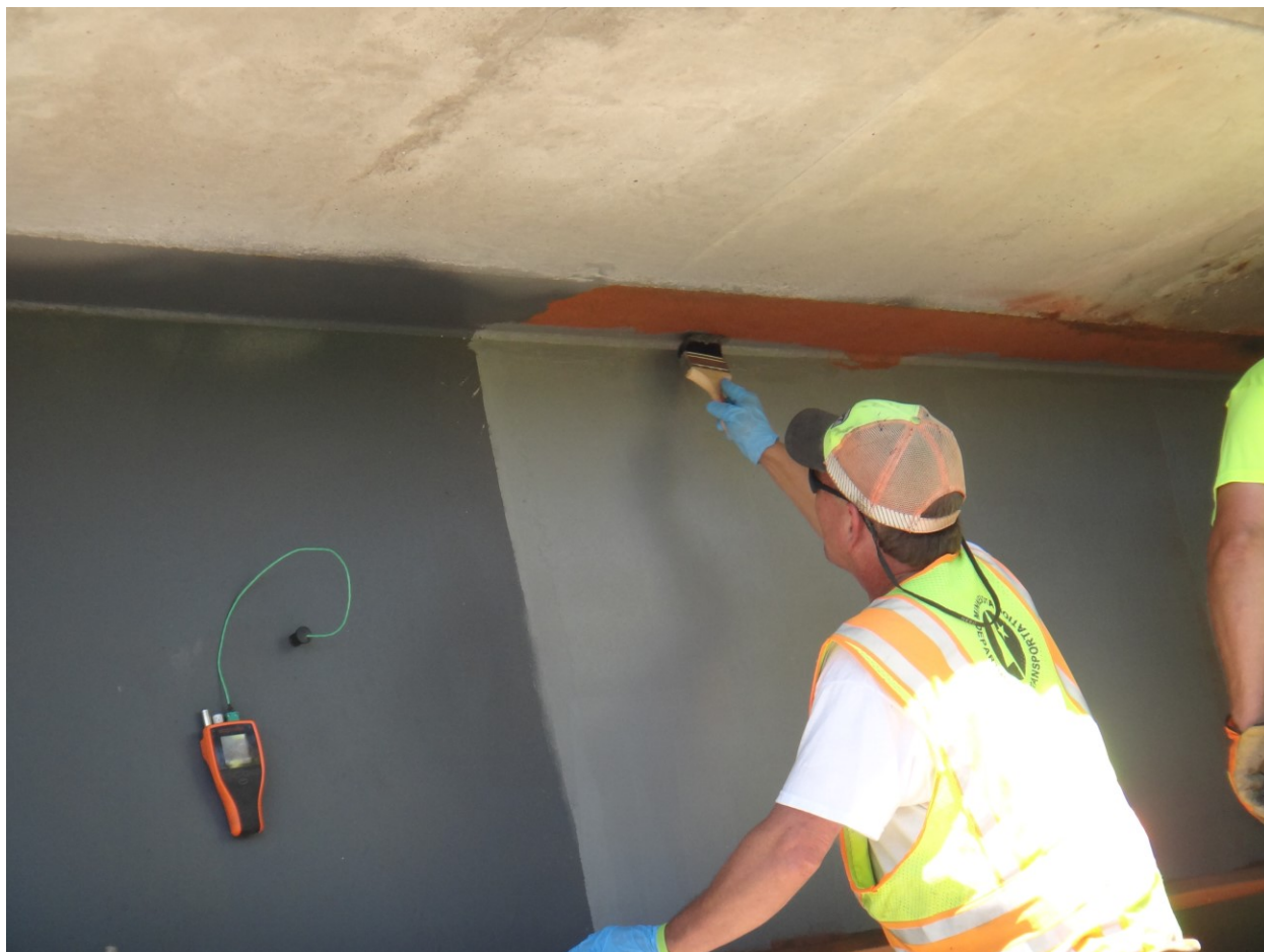
Figure 4.12 Test Location 3 Prime Coat Application
