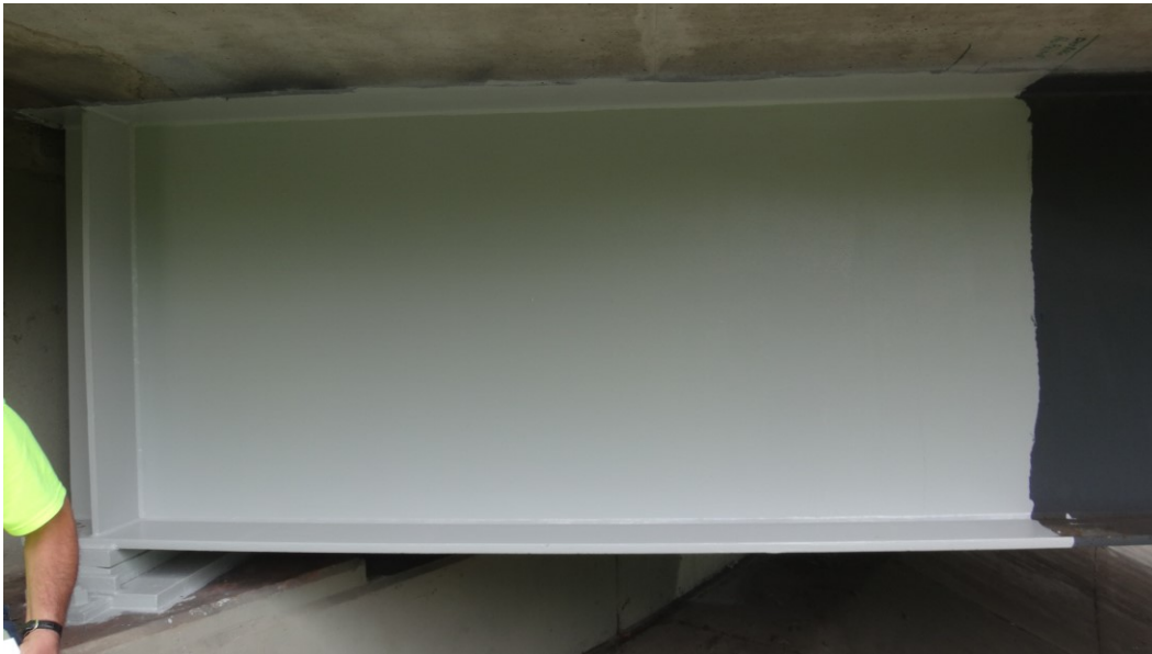
Figure 4.18 Test Location 4 Finish Coat
