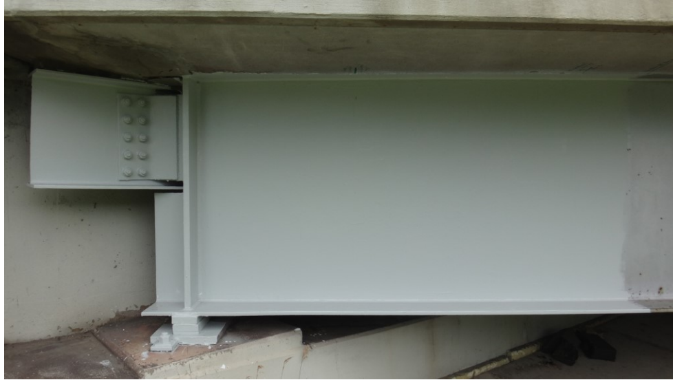
Figure 4.19 Test Location5 Finish Coat
