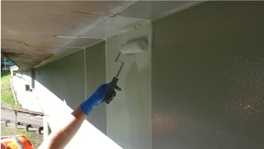
Figure 8.9 Additional Test Patch Location D - Coating Application
