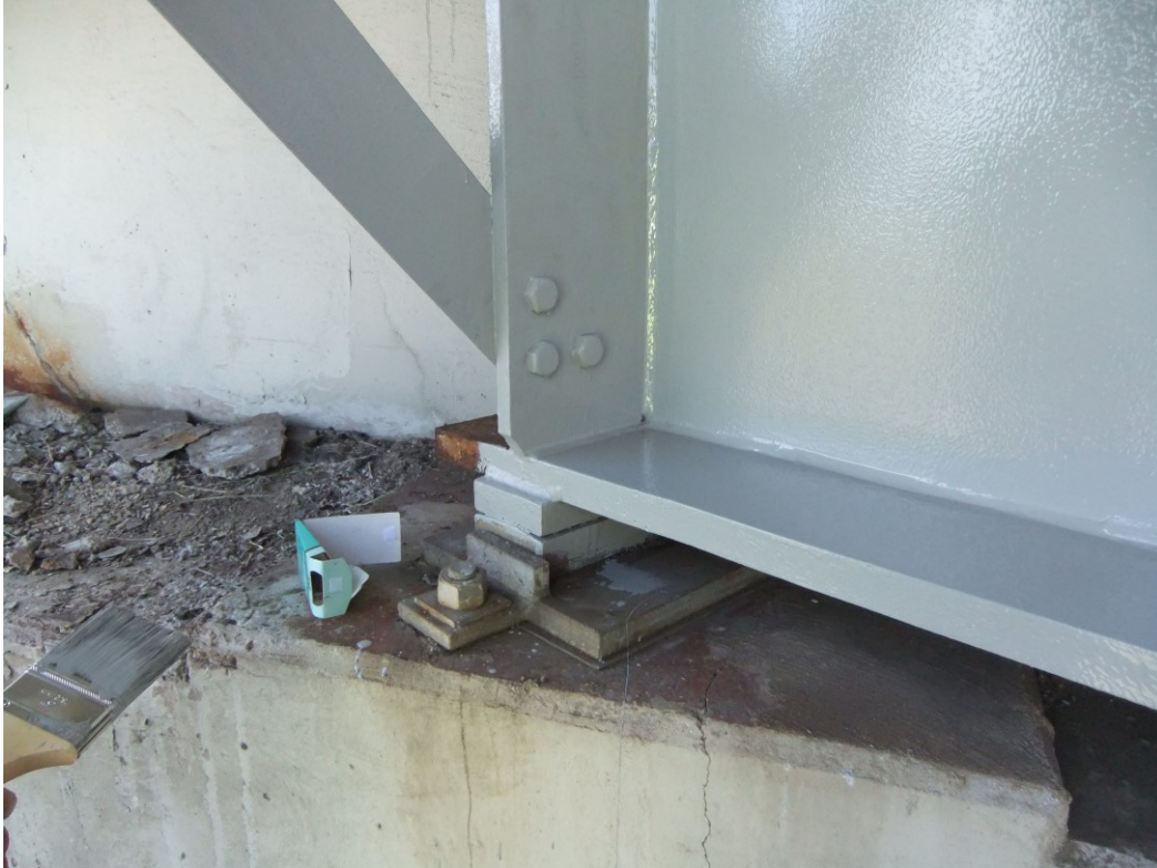
Figure 4.11 Test Location 2 Prime Coat Application
