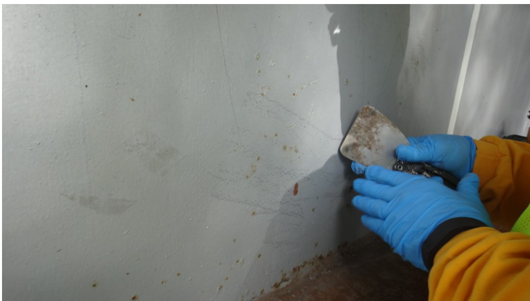
Figure 8.4 Additional Test Patch Locations – SP2 Hand Tool Clean Surface Preparation
