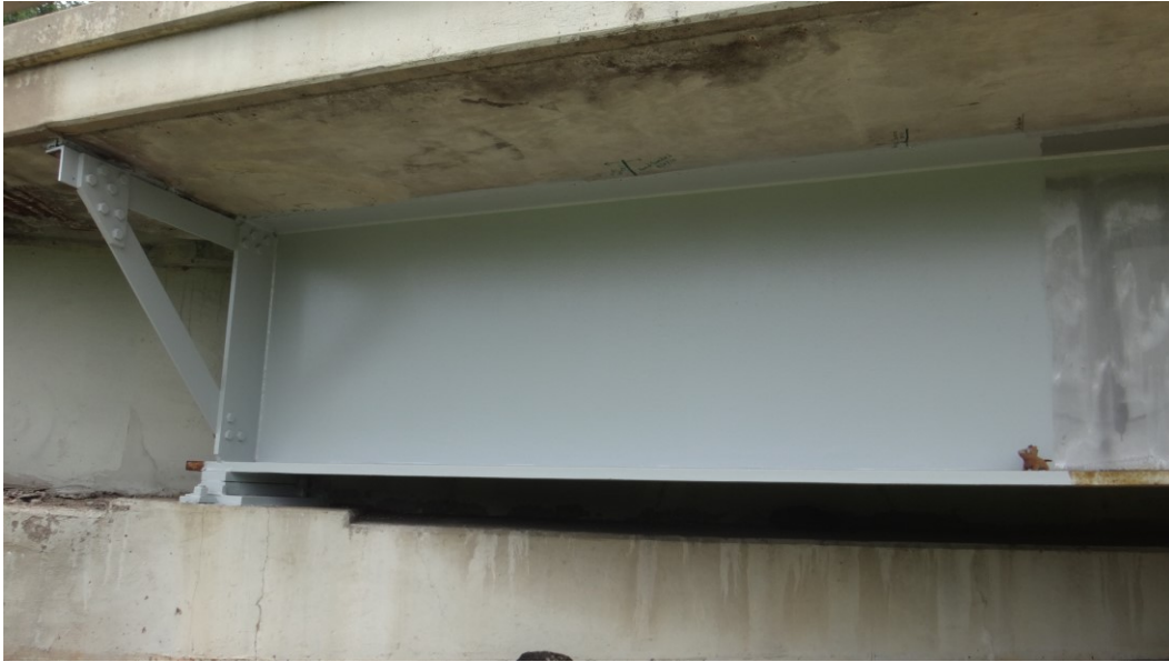
Figure 4.16 Test Location 2 Finish Coat
