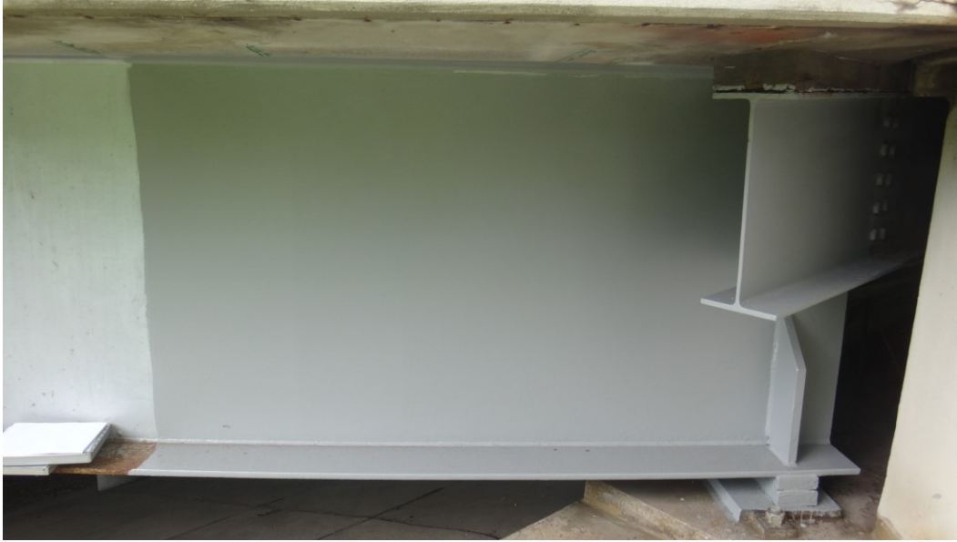
Figure 4.15 Test Location 1 Finish Coat
