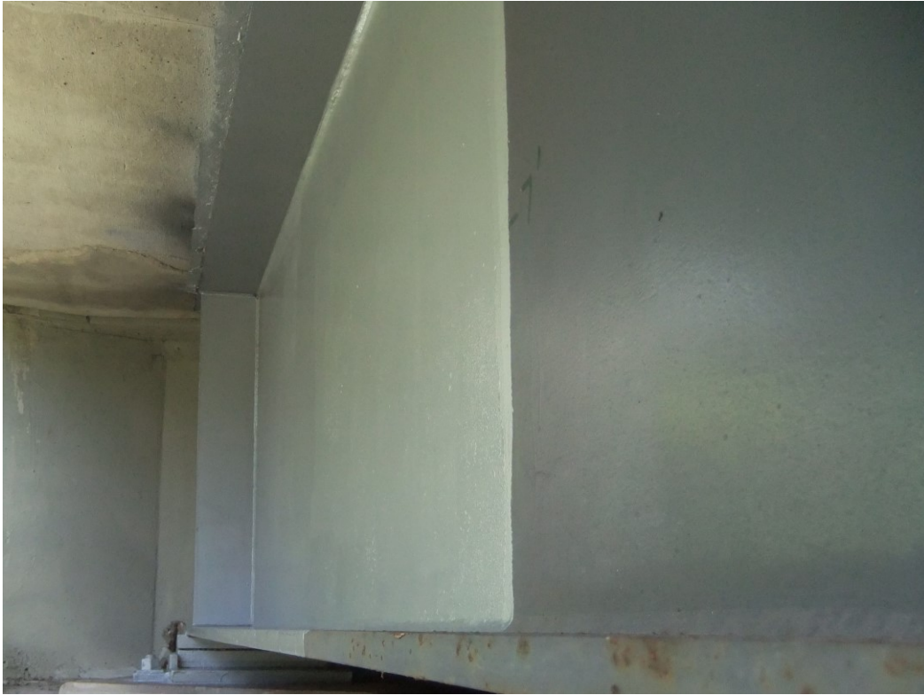
Figure 4.13 Test Location 4 Prime Coat Application
