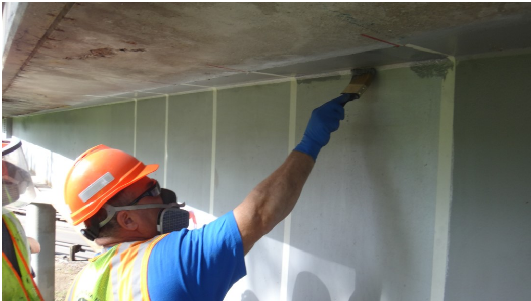
Figure 8.6 Additional Test Patch Location A - Coating Application
