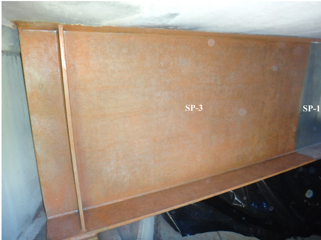
Figure 4.8 Test Location 4 Surface Preparation
