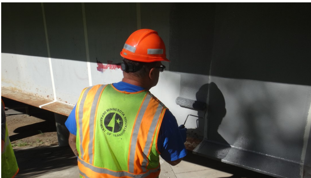
Figure 8.7 Additional Test Patch Location B - Coating Application
