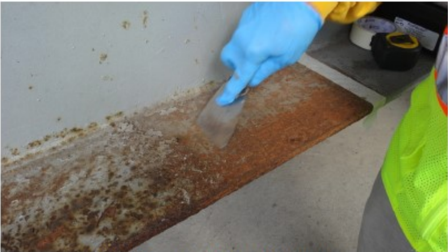
Surface Prep Spot SP2 at Bottom Flange
