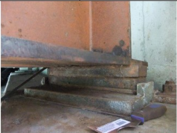
Surface Prep (2) (Removed Anti-Graffiti Coating with Power Tools)
