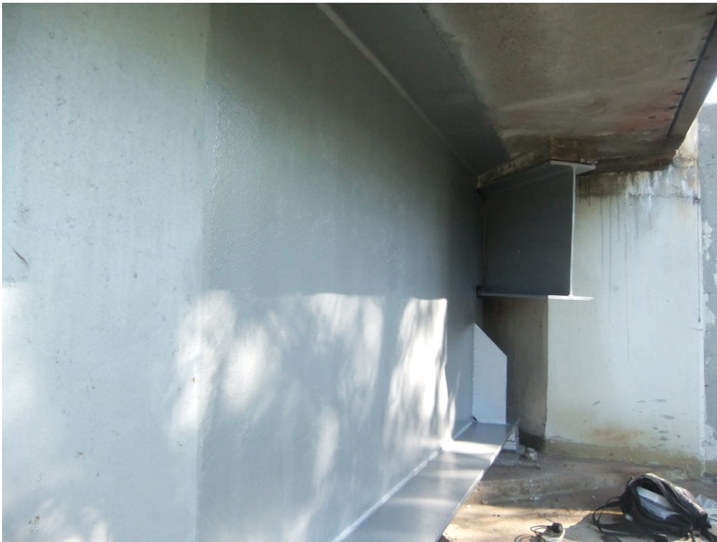
Figure 4.10 Test Location 1 Prime Coat Application
