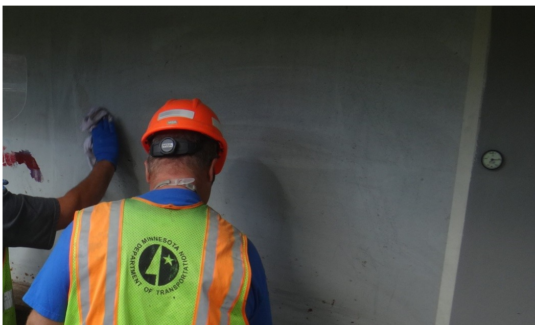
Figure 8.5 Additional Test Patch Locations – SP1 Solvent Clean Surface Preparation Employing a Dry Rag
