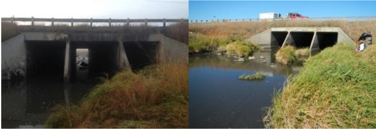
Figure 2.4 Upstream view of culvert 91077 on Elk Creek, Rock County, showing a portion of the small pool (left) and downstream view of culvert 91077, showing vegetated islands and rip-rapped area.
