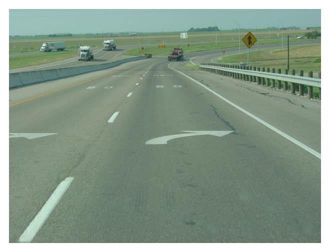
Figure 3.19 Urban freeway curve warning pavement markings (39).
