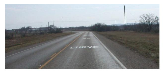
Figure 3.18 Text and advisory speed horizontal signing applications (39).
