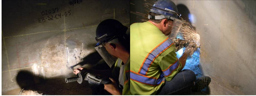
Figure 3.6. (Left) Exposing post-tensioning duct by cutting web
