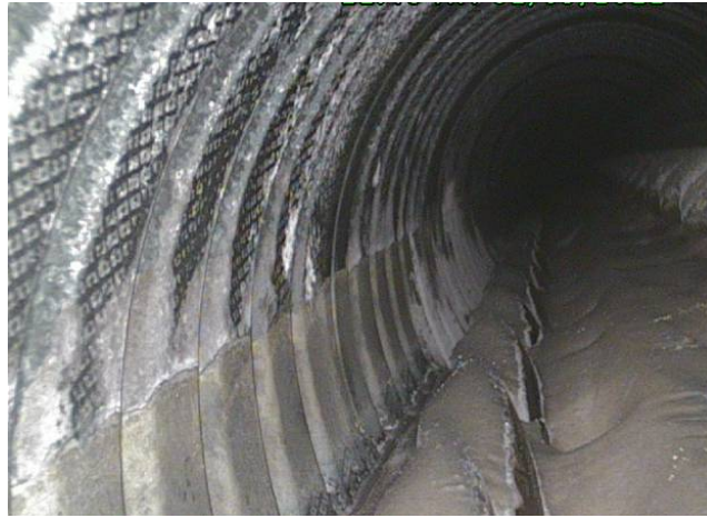
Figure 8.21. Borescope picture looking toward highpoint in tendon 3, 24 inches (61 centimeters) inside of the inspection hole
