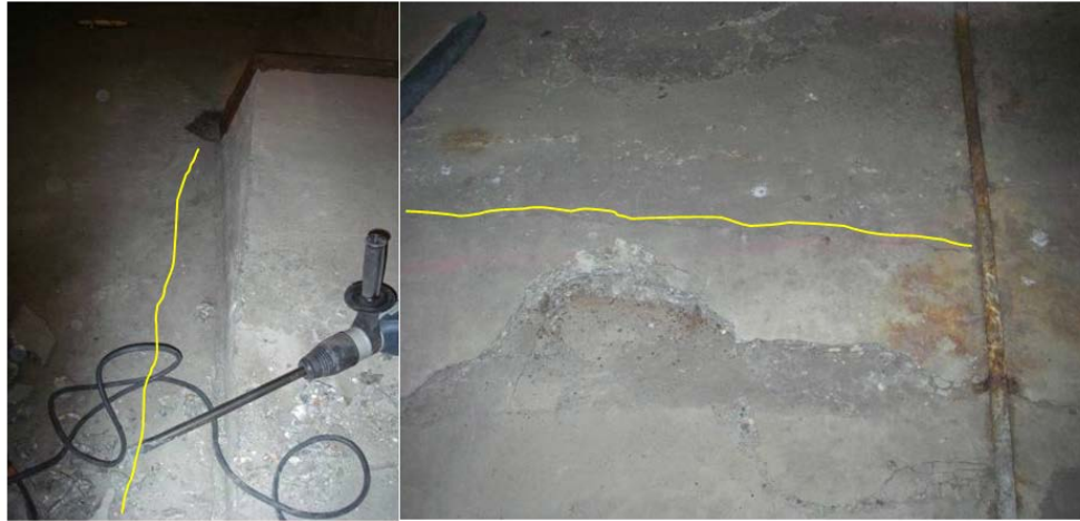
Figure 6.27. (Left) Crack along anchorage of tendon B28/B24
