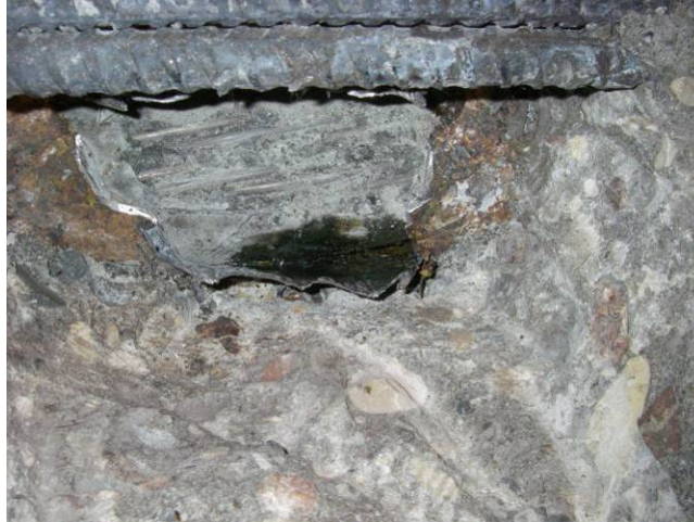
Figure 6.25. Opened tendon 16 with green corrosion product
