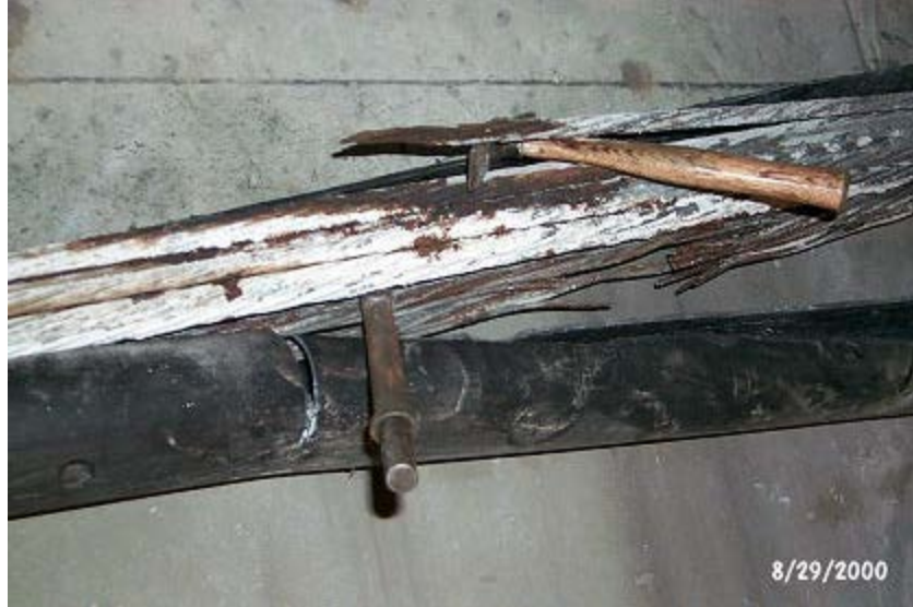
Figure 2.5. Corroded tendons at breached duct (Corven Engineering, 2002)
