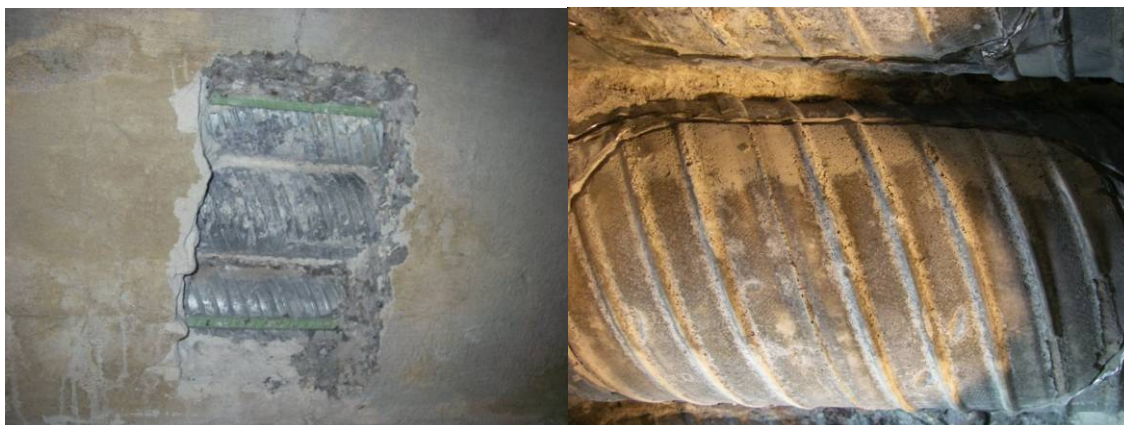
Figure 8.3. (Left) Cut out area exposing ducts
