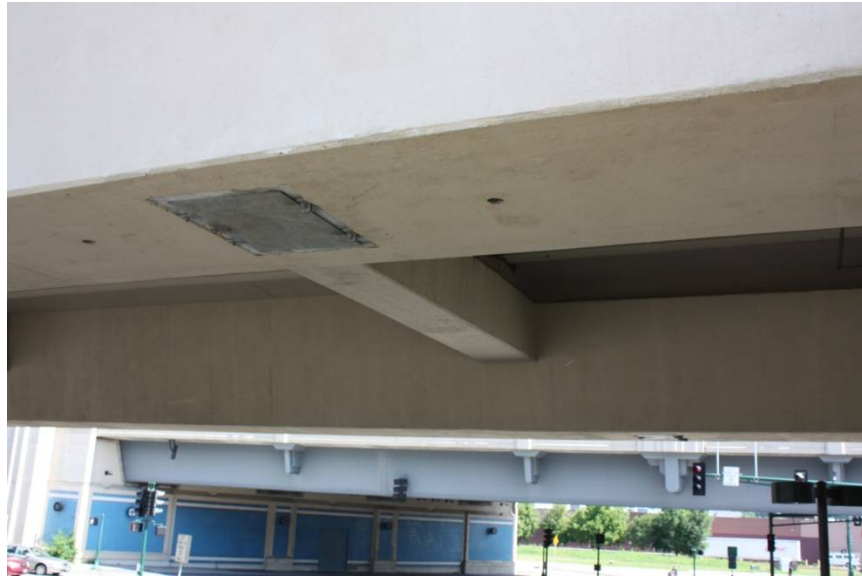
Figure 5.2. Access hatch of bridge 27262
