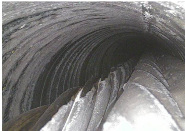
Figure 8.20. Borescope picture looking toward highpoint in tendon 3, 6 inches (15.2 centimeters) inside of the inspection hole
