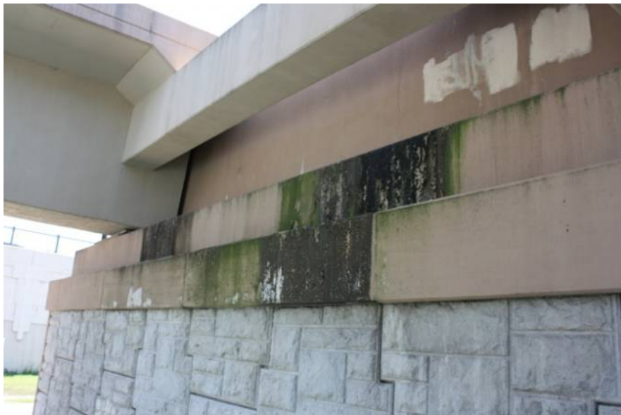
Figure 5.3. Discoloration of abutment
