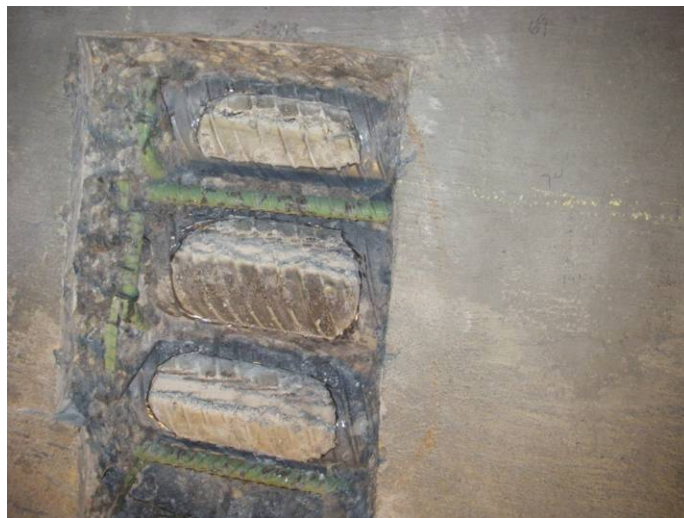
Figure 8.6. Exposed ducts in girder 5 of span 2
