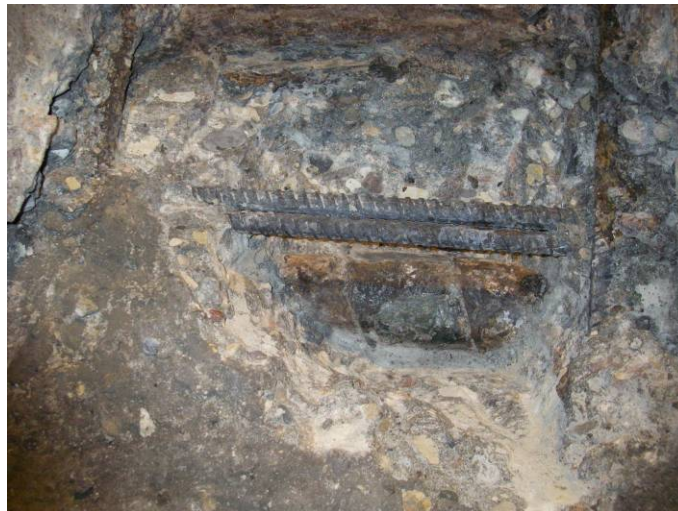
Figure 6.24. Shows tendon 16 with corroded duct
