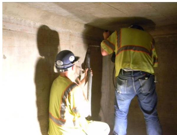
Figure 3.2. Drilling into post-tensioning duct
