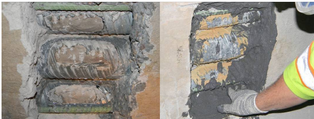
Figure 3.8. (Left) Exposed post-tensioning strand
