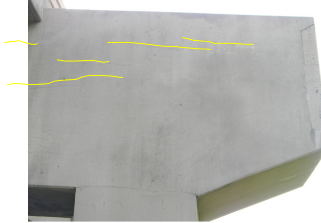
Figure 10.2. Cracking along straddle bent
