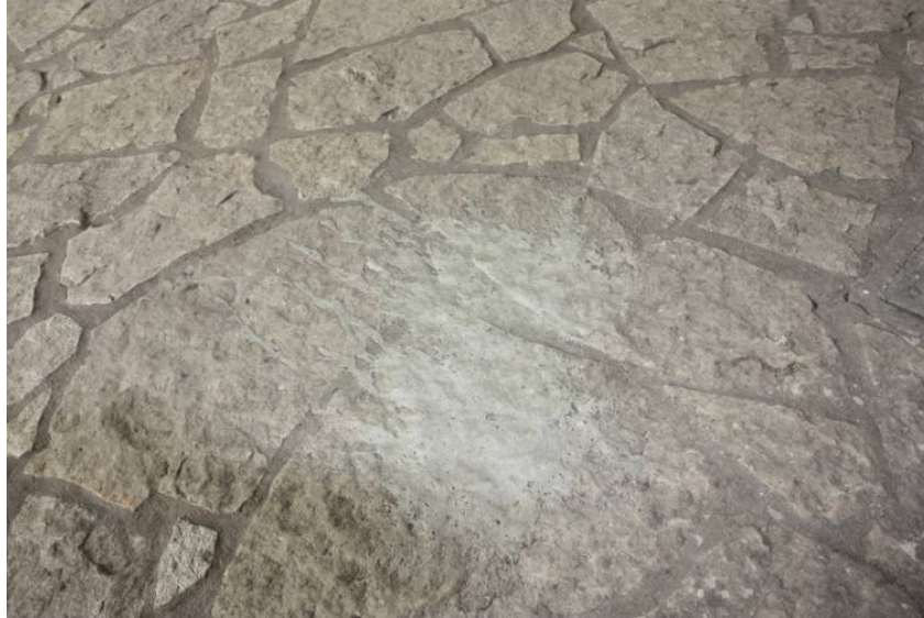
Figure 5.8. Grout splatter beneath access hatch
