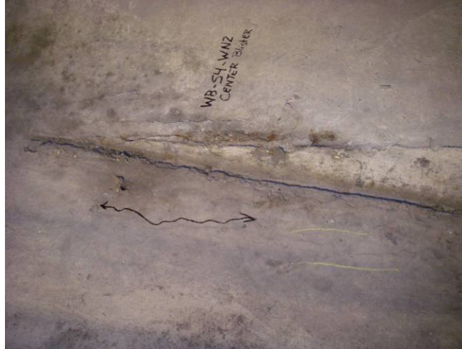
Figure 6.36. Cracking along anchorage blister in span 4
