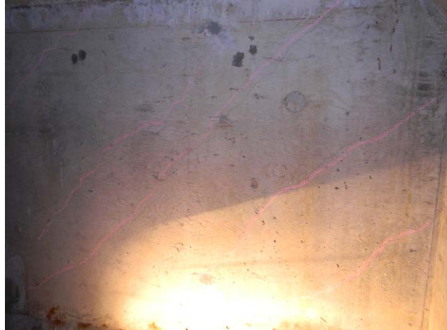
Figure 7.8. Diagonal cracking on interior of box girder
