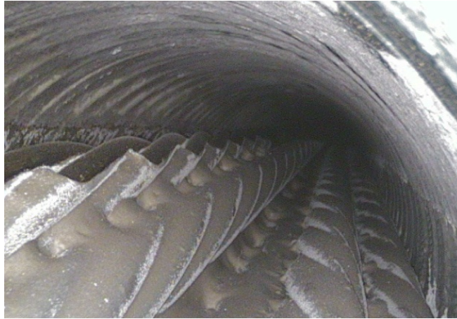
Figure 8.23. Borescope picture looking toward low point in tendon 3, 6 inches (15.2 centimeters) inside of the inspection hole
