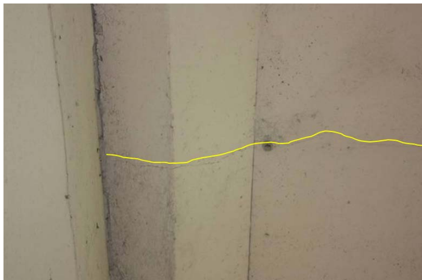
Figure 5.9. Cracking along box girder
