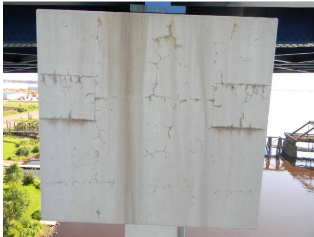
Figure 9.1. PT cap on Blatnick Bridge pier
