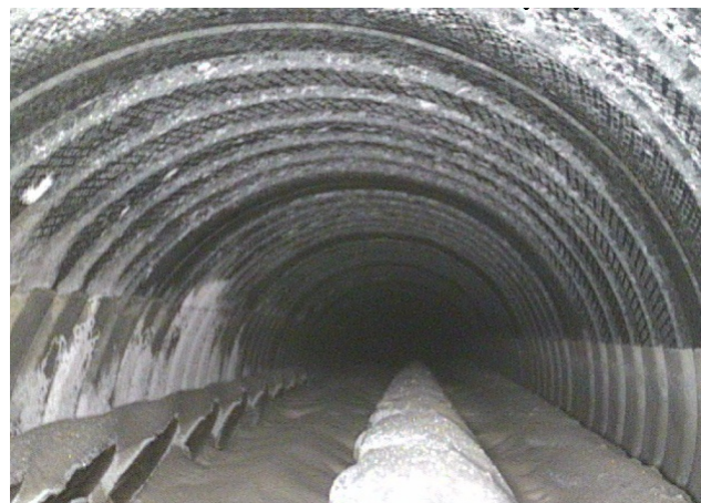
Figure 8.22. Borescope picture looking toward highpoint in tendon 3, 3.5 feet (1.07 meters) inside of the inspection hole
