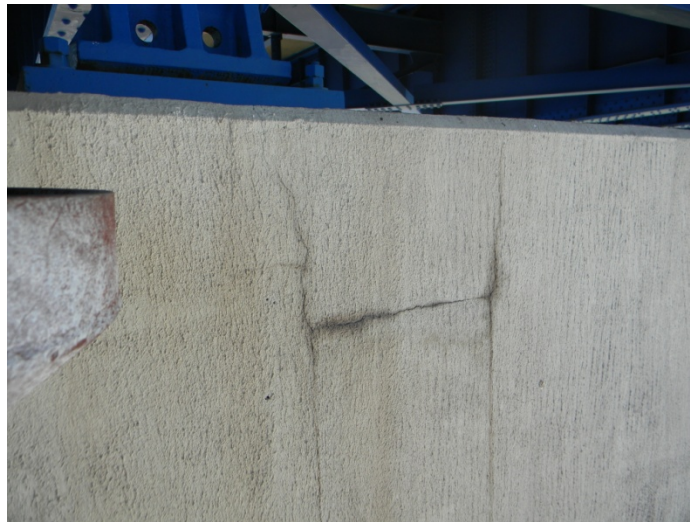
Figure 9.3. Vertical and horizontal cracking in pier
