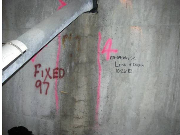
Figure 6.34. Drainage duct with moisture staining
