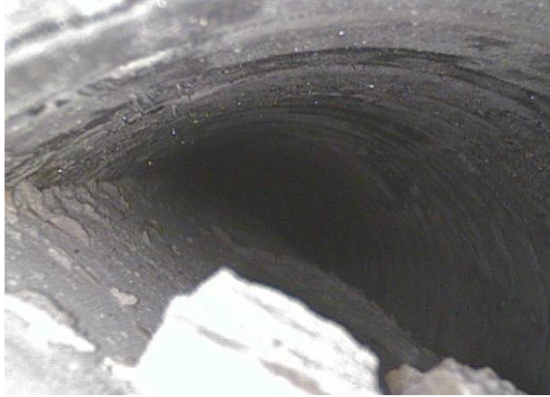
Figure 8.14. Borescope picture looking toward highpoint in tendon 3
