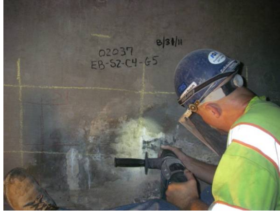
Figure 8.5. Removing cover at inspection area
