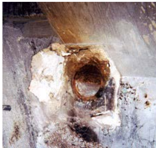
Figure 2.3. Water staining at expansion joint around anchor where tendon corroded (Corven Engineering, 2002)
