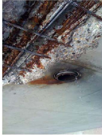
Figure 6.4. Bottom slab drainage outlet (Corven Engineering, 2010)
