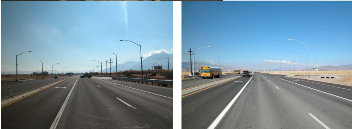
FIGURE 4-5 US 395 Turn Lanes on the North (left photo) and South (right photo) Approaches
