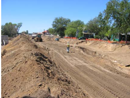
Figure 2.1. Construction of Highway 10 in Staples, MN.
