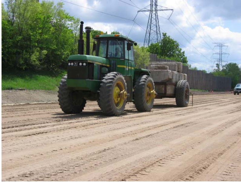
Figure 1.3. Test rolling a compacted subgrade.
