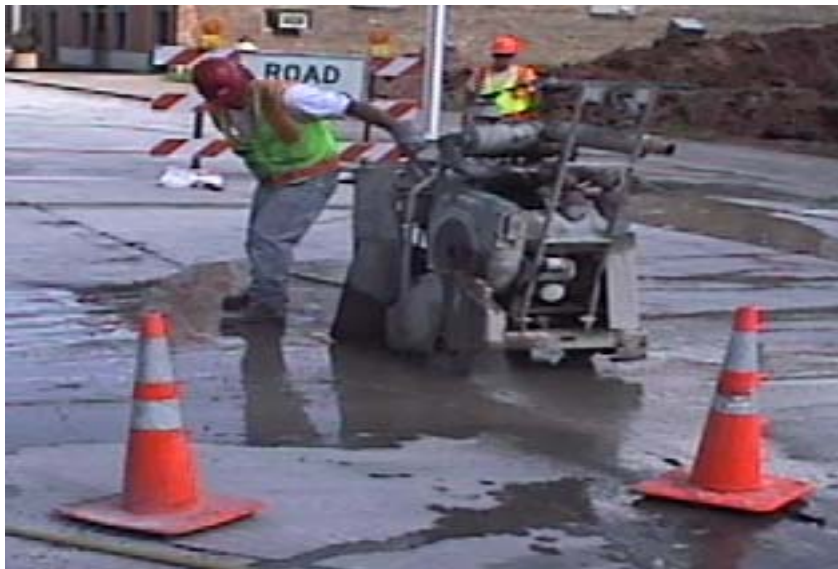
Figure 3.1 Sawing of joint before re-sealing.
