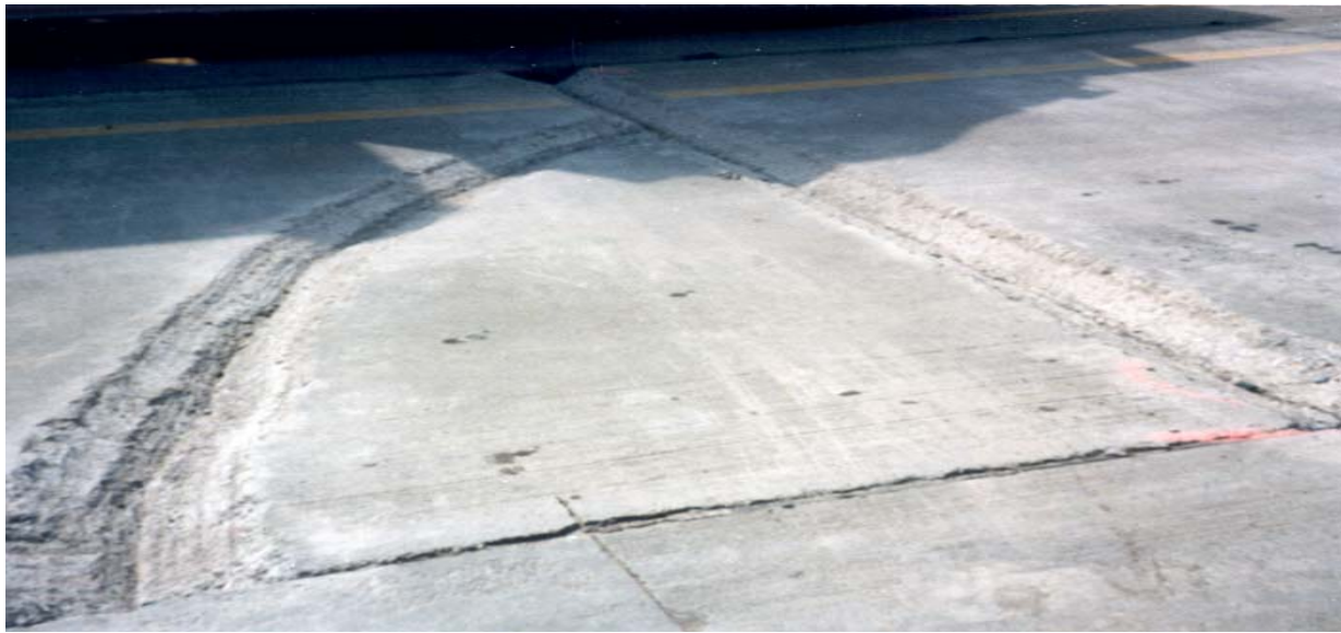
Figure 4.1 View of partial depth repairs after milling operations, both a joint and a crack.
